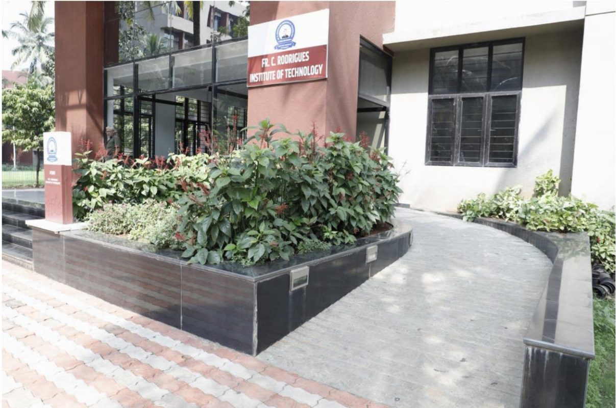
RAMP FOR DIFFERENTLY ABLED
